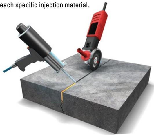
**Gravitational filling:** Gravitational filling is performed under pressureless conditions (and without packers). Wide cracks can be filled without preparation, whereas narrow cracks will need to be ground out first.
